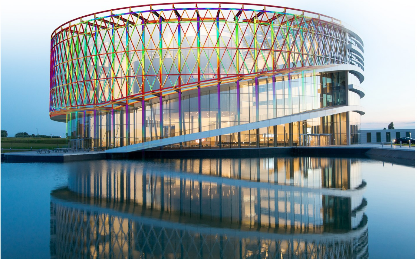
Barco One Campus - © Image Jaspers-Eyers Architects – photography by Marc Detiffe
